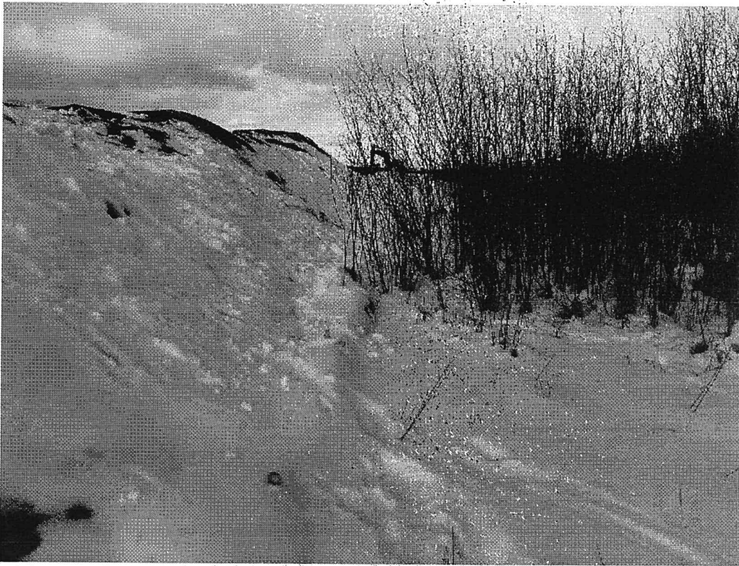
Photo 7 – Photo Point 6. View northeast of leachfield mound fill adjacent to and likely into surface water/wetland complex (November 16, 2022).
