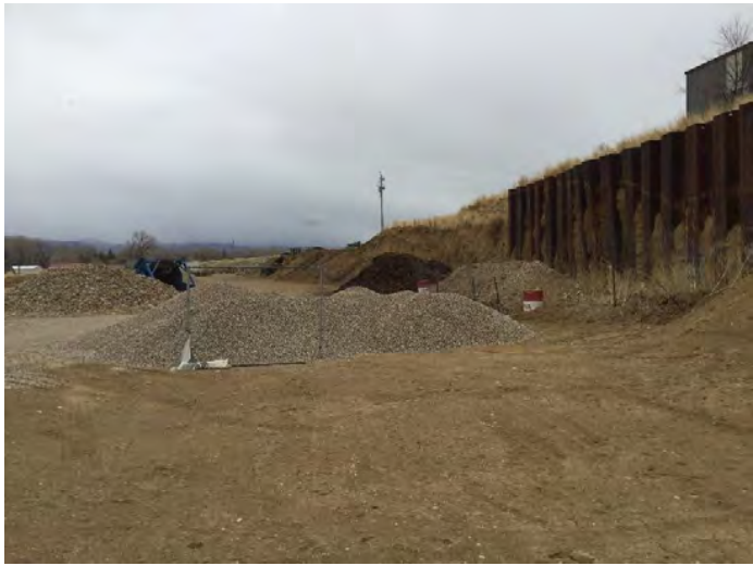
Photo #7: Materials stockpiled against the highwall on the south side of the LMO boundary. The stockpiled material has decreased in volume. Photo taken May 27, 2021.
