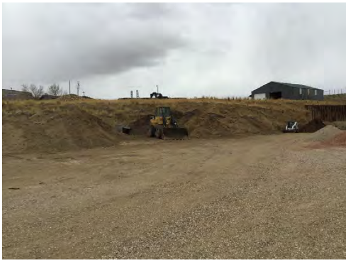
Photo #5: Materials stockpiled against the highwall on the south side of the LMO boundary. The stockpiled material has decreased in volume. Photo taken May 27, 2021.
