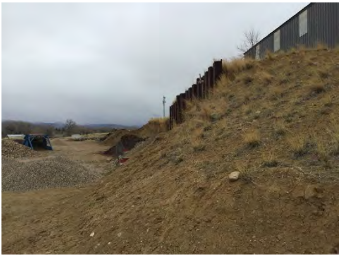
Photo #6: Materials stockpiled against the highwall on the south side of the LMO boundary. The stockpiled material has decreased in volume. Photo taken May 27, 2021.
