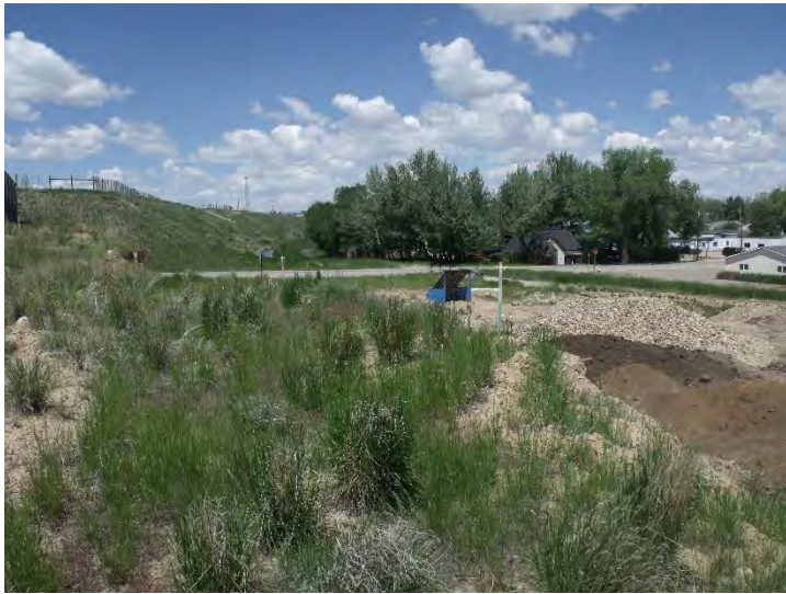
Photo #4: General overview of the top of the steel retaining wall and LMO boundary. Mining has occurred outside the LMO legal description.
