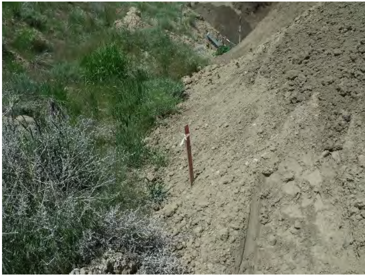
Photo #2: General overview of survey markers place on the southern LMO boundary. Material stockpiles are being placed on top the survey markers and outside the LMO legal description.
