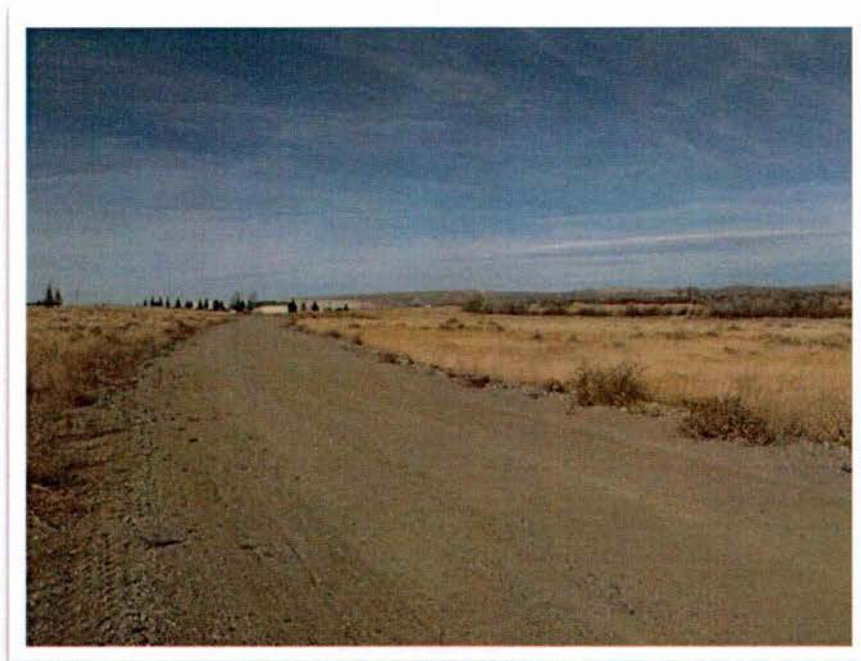
Photo #5: Constructed road at the 10 acre tract of land.
