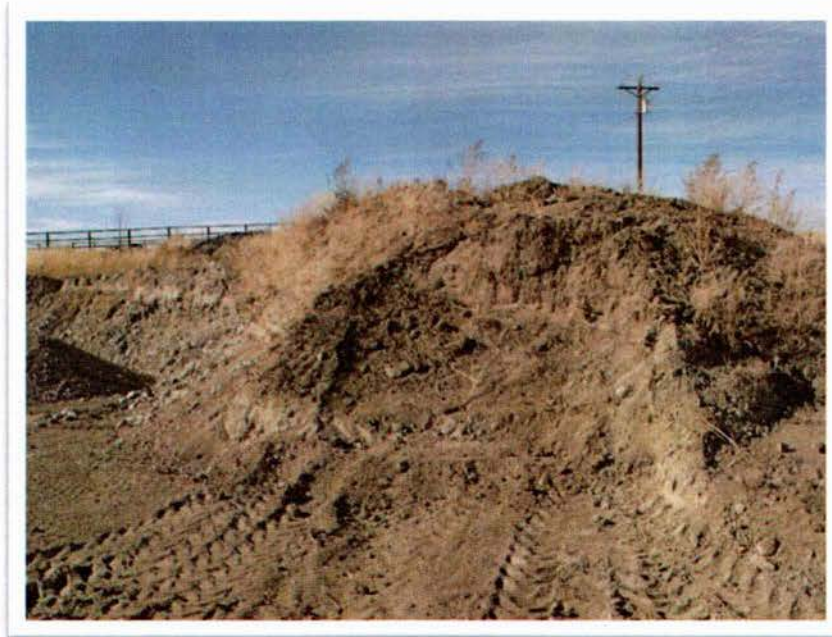
Photo #1: Topsoil and subsoil stockpiled at 10 acre tract of land.
