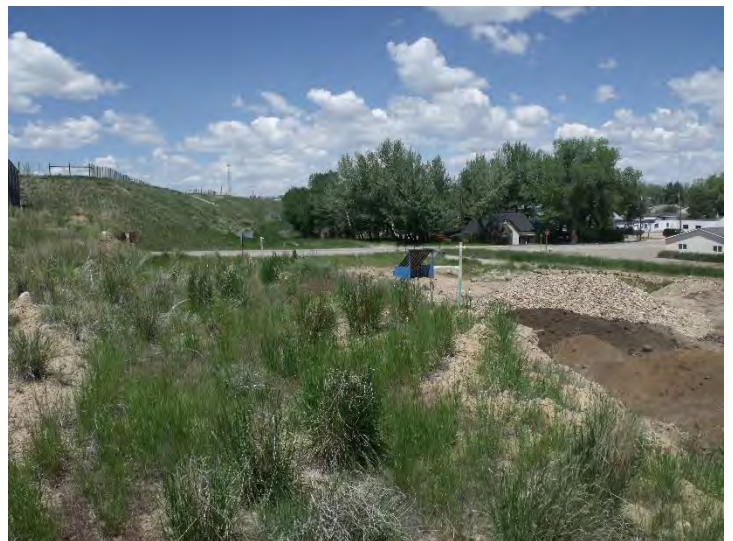
Photo #4: General overview of the top of the steel retaining wall and LMO boundary. Mining has occurred outside the LMO legal description.
