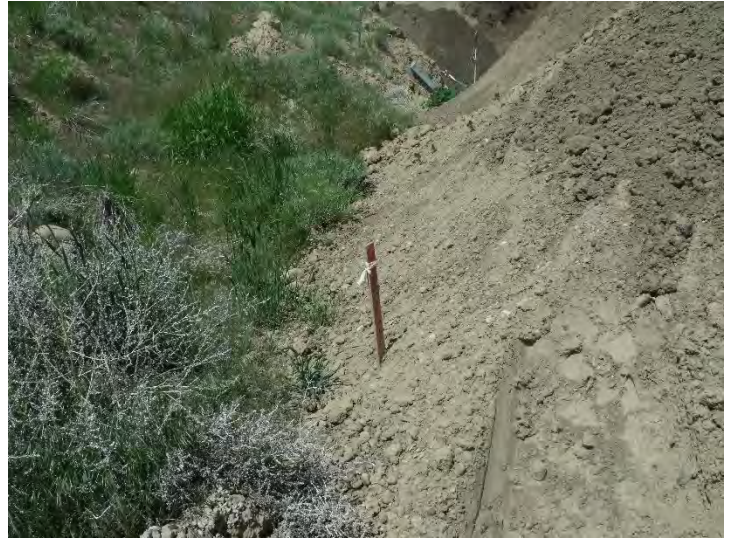
Photo #2: General overview of survey markers placed on the southern LMO boundary. Material stockpiles are being placed on top of the survey markers and outside the LMO legal description.
