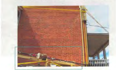
Steel Cables Around the House
