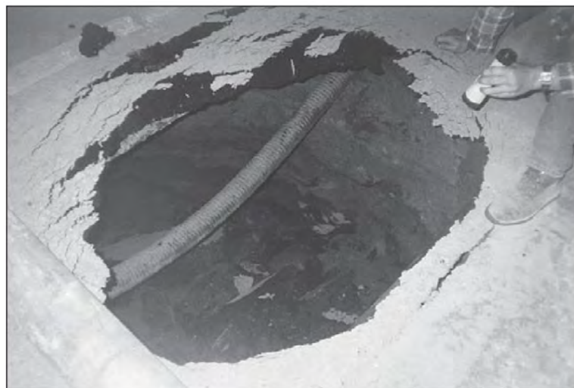
Fig 2.2.2 Subsidence hole (Crowell 2010)
