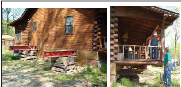
Plywood placed around foundation to keep home warmer over the winter
