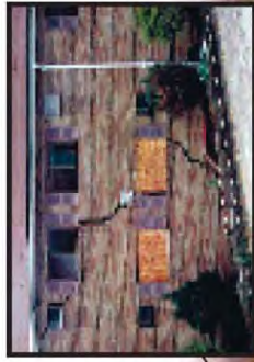
Illustration of Trough Subsidence.
