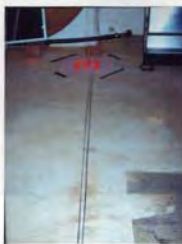
Slot in Concrete
