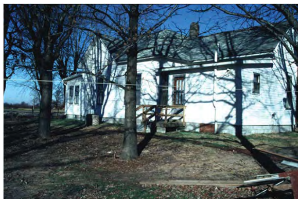
Reset several months after pass of longwall
