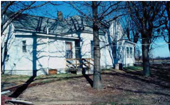
Home reset on new foundation after completion of subsidence movements
