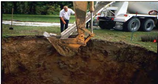
Fill the Sinkhole with Concrete
