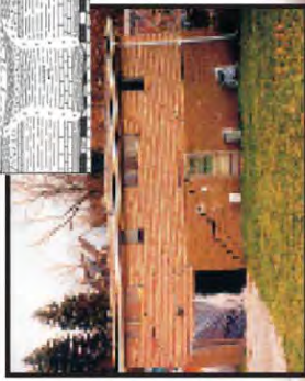
Illustration of Trough Subsidence.
