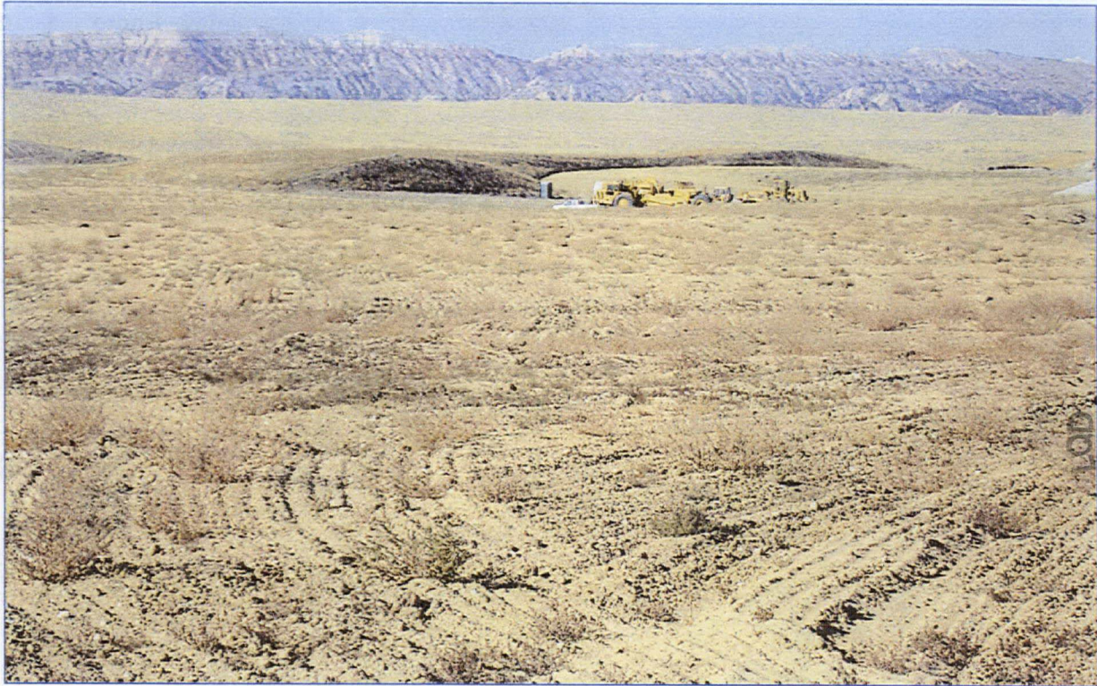
Photo 3 (top) looks south-southwest and shows a regraded hill of suitable material. The hill may or may not stay as a feature on the reclaimed landscape; its fate will be dependent on cover material needs. The foreground shows the vegetation present in the 2011 seeding, which is dominated by Russian Thistle and Halogeton. Photo 4 (bottom) looks east and shows the vegetative condition of a portion of the potential mine area located east of Bear Creek.
