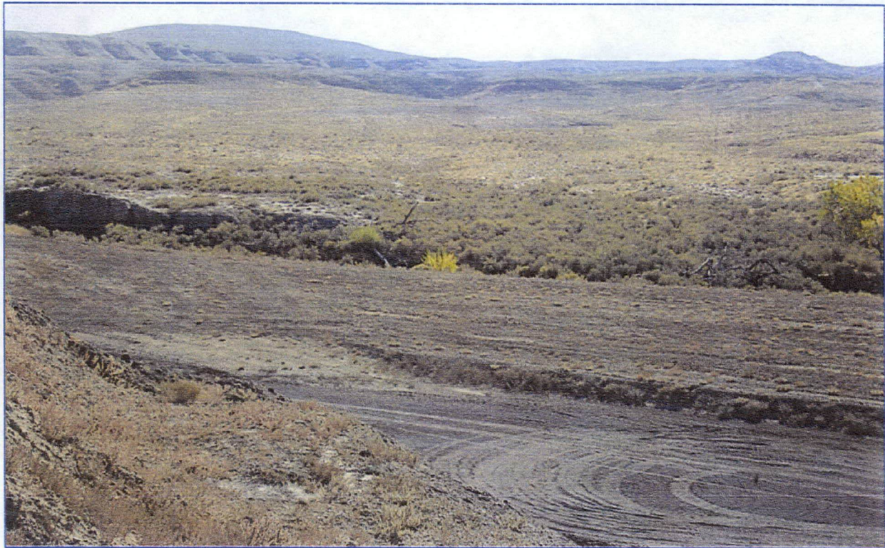
Photo 3 (top) looks south-southwest and shows a regraded hill of suitable material. The hill may or may not stay as a feature on the reclaimed landscape; its fate will be dependent on cover material needs. The foreground shows the vegetation present in the 2011 seeding, which is dominated by Russian Thistle and Halogeton. Photo 4 (bottom) looks east and shows the vegetative condition of a portion of the potential mine area located east of Bear Creek.
