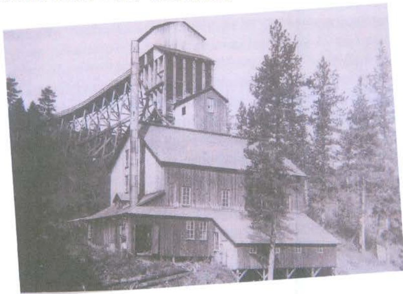
The Inter Ocean Mill as it appeared in 1903. The facility housed a 20-stamp mill and was constructed to process ore brought by tramway from the Inter Ocean Mine.
