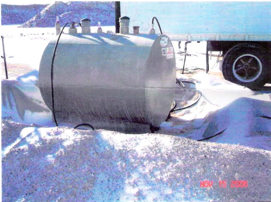
Photo 1: Fuel tank used for the screen that is located in a bermed area with a plastic liner. MCC has been asked to increase the size of the berm on the right provide added protection.
