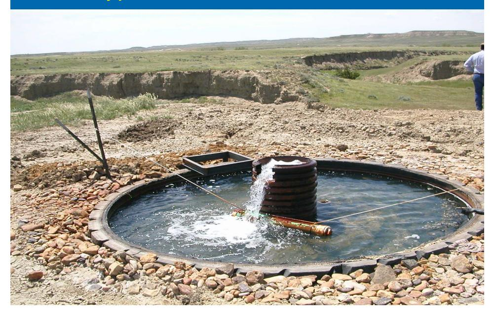
There Are About 4,000 Constructed CBM Outfalls. Most are in the Powder River Basin
