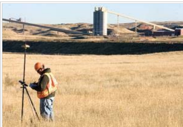
Paul Guajardo, a surveyor for Ames Construction, records positions for a power block that will accompany the new Dry Fork Station power plant. The 385-megawatt plant construction began Wednesday north of Gillette near the mouth of the Dry Fork mine. — News-Record photo by Nathan Payne
