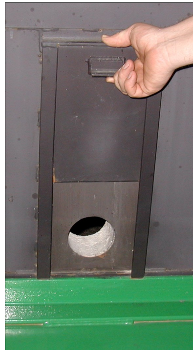
Access Door for Lighting
