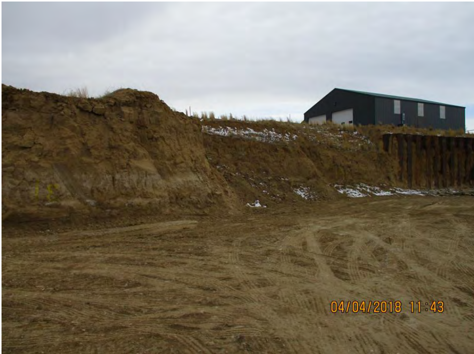
Picture taken by State Mine Inspector 4/4/2018
