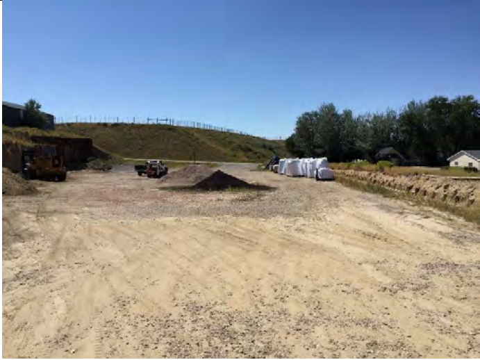
Photo #12: QLN constructed commercial access to the LMO. Photo taken August 8, 2022
