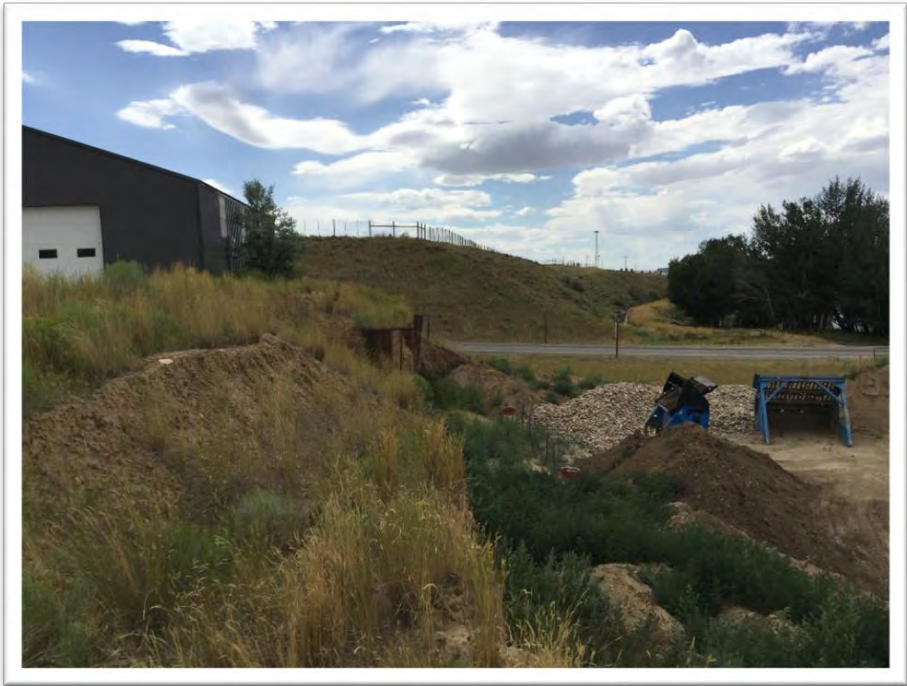
Photo #9: Mining has occurred outside the legal description and has resulted in material damage to steel retaining wall and adjacent property. Photo taken on July 14, 2020.
