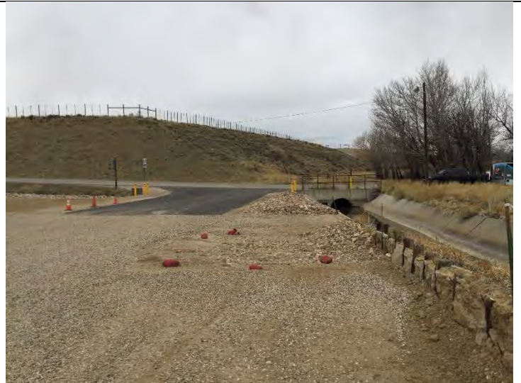
Photo #12: QLN constructed commercial access to the LMO.
