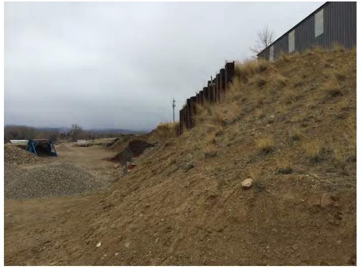
Photo #6: Materials stockpiled against the highwall on the south side of the LMO boundary. The stockpiled material has decreased in volume. Photo taken May 27, 2021.
