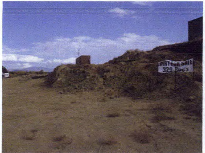
Photo #4: General overview of highwall looking east direction. Steel wall installed to stabilize the slope.
