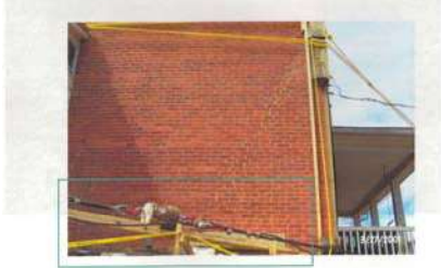
Steel Cables Around the House
