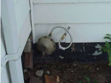
Utility precautions during subsidence
