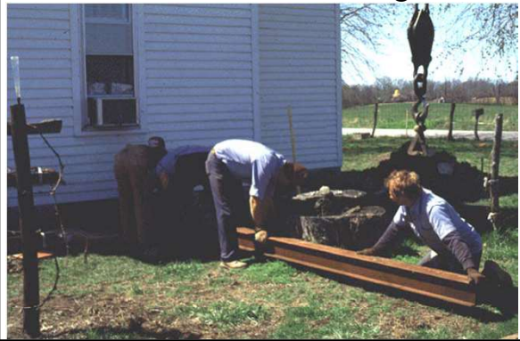
“I” Beams for Floating
