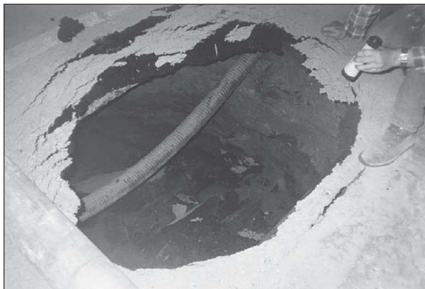
Fig 2.2.2 Subsidence hole (Crowell 2010)
