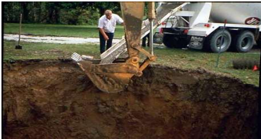
Fill the Sinkhole with Concrete
