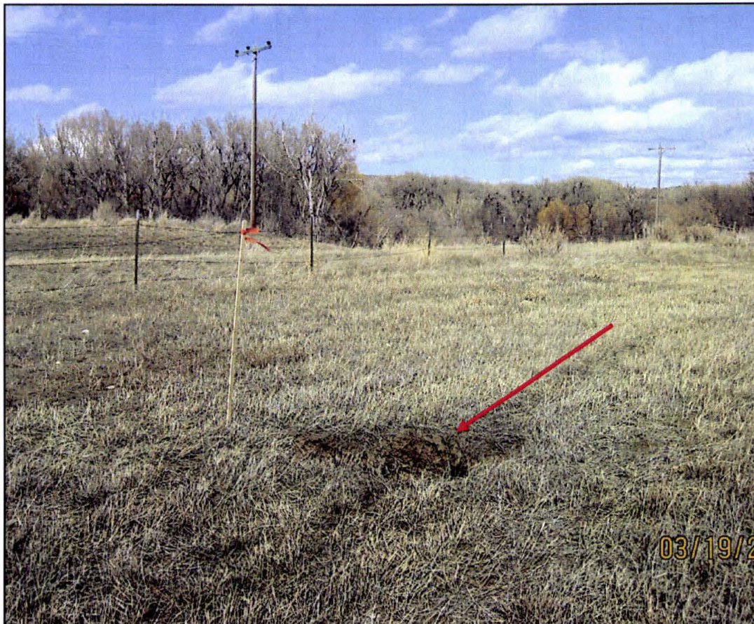
Old Monarch subsidence, open to workings.
