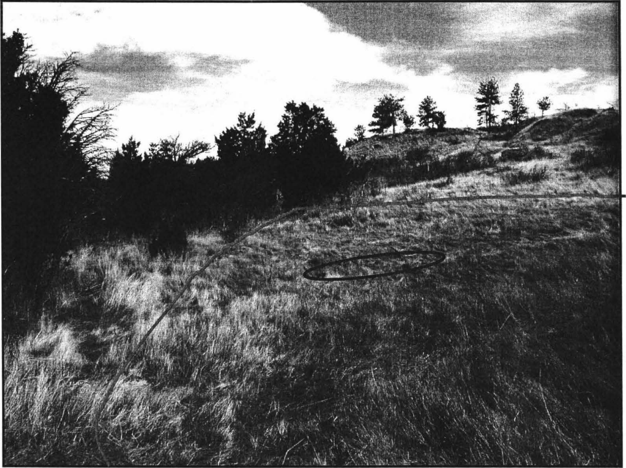
Photo 5: Borrow area should remain inside blue line. Red oval denotes subsidence location.
