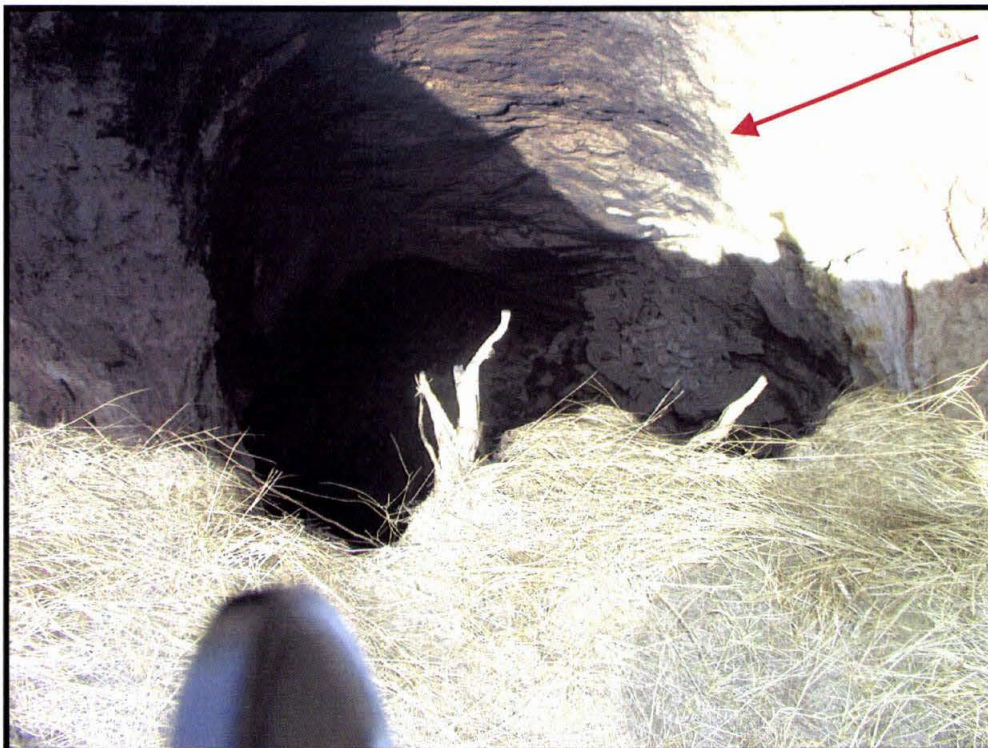
Photo 4: Looking into bottom of fire subsidence vent hole. Note smoke residue/coal tar deposit on wall where smoke chimneys up the side. Note opening in bottom leading to voids.
