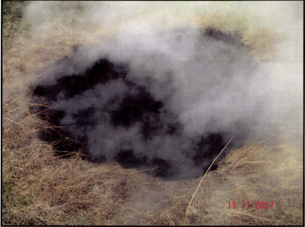
Photo 2: Open subsidence hole. Approximate depth 25-30 feet, diameter approximately 8-10 feet.
