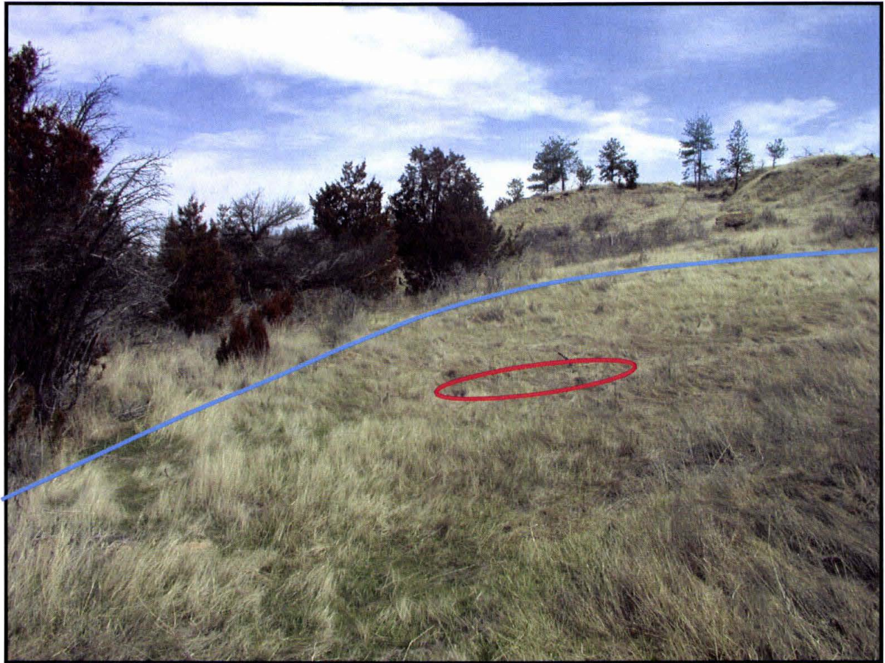
Photo 5: Blue line indicates division between native and previously disturbed area. Red oval denotes subsidence location.
