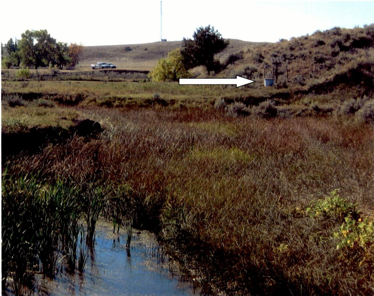
Stilling well on right bank of Slater Creek, observed during September 23, 2015 site visit. Site was believed to be station SM578512-SW-1. Approximate location of this site is shown in the map below.
