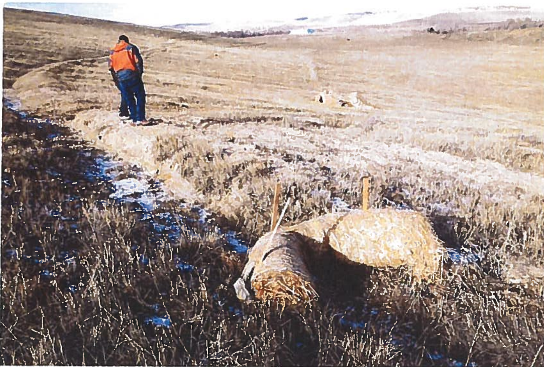
Photo 3: (north) erosion control measures put in place to protect repair and reseeding
