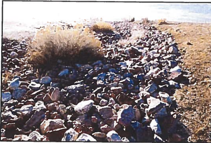
Photo 4: (southeast) looking downstream on the drainage leading to pit 3 reservoir (erosion controls functioning)
