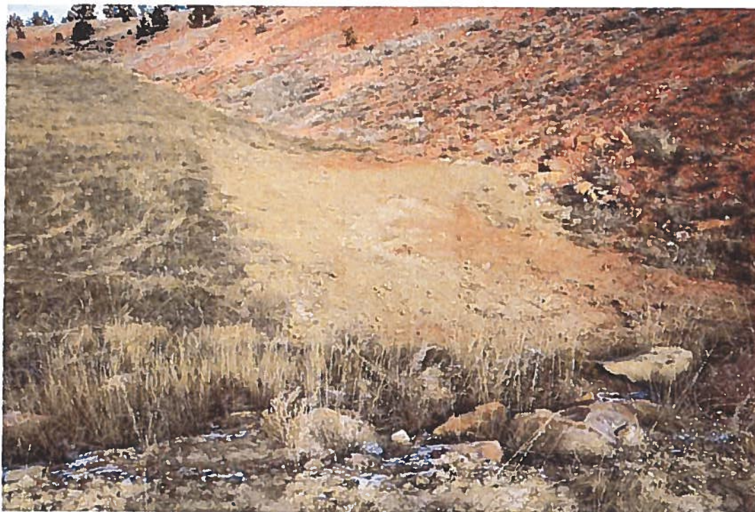
Photo 4: (south) repairs and reseeding at solid waste disposal area
