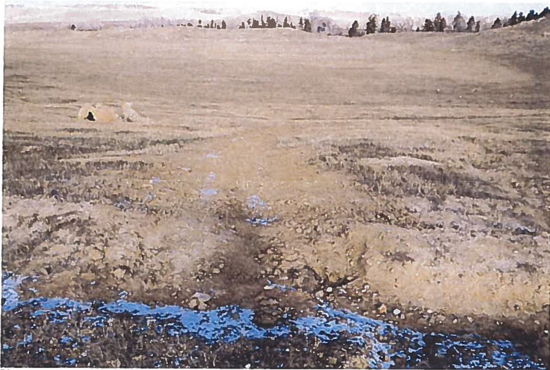
Photo 2: (northwest) repairs and reseeded on gullied areas
