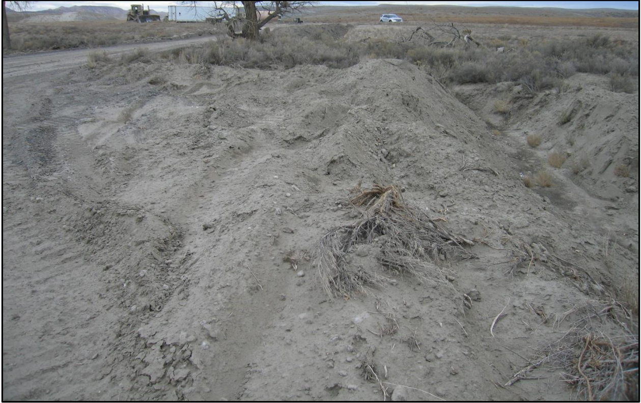
Photo 7 (above) looks west at an area of orphaned topsoil that pushed up near the northwest corner of the East Pit. To avoid contamination this material should either be placed in a stockpile or picked and “live spread” during the next sub / top soil respreads effort. Photo 8 (below) looks south across the recently reclaimed area immediately east of Bear Creek. The bentonite stockpile in the background is associated with WDEQ/LQD Permit 278.
