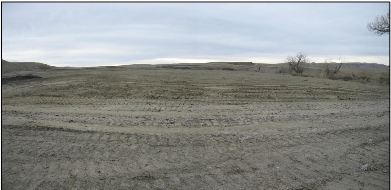
Photo 7 (above) looks west at an area of orphaned topsoil that pushed up near the northwest corner of the East Pit. To avoid contamination this material should either be placed in a stockpile or picked and “live spread” during the next sub / top soil respreads effort. Photo 8 (below) looks south across the recently reclaimed area immediately east of Bear Creek. The bentonite stockpile in the background is associated with WDEQ/LQD Permit 278.
