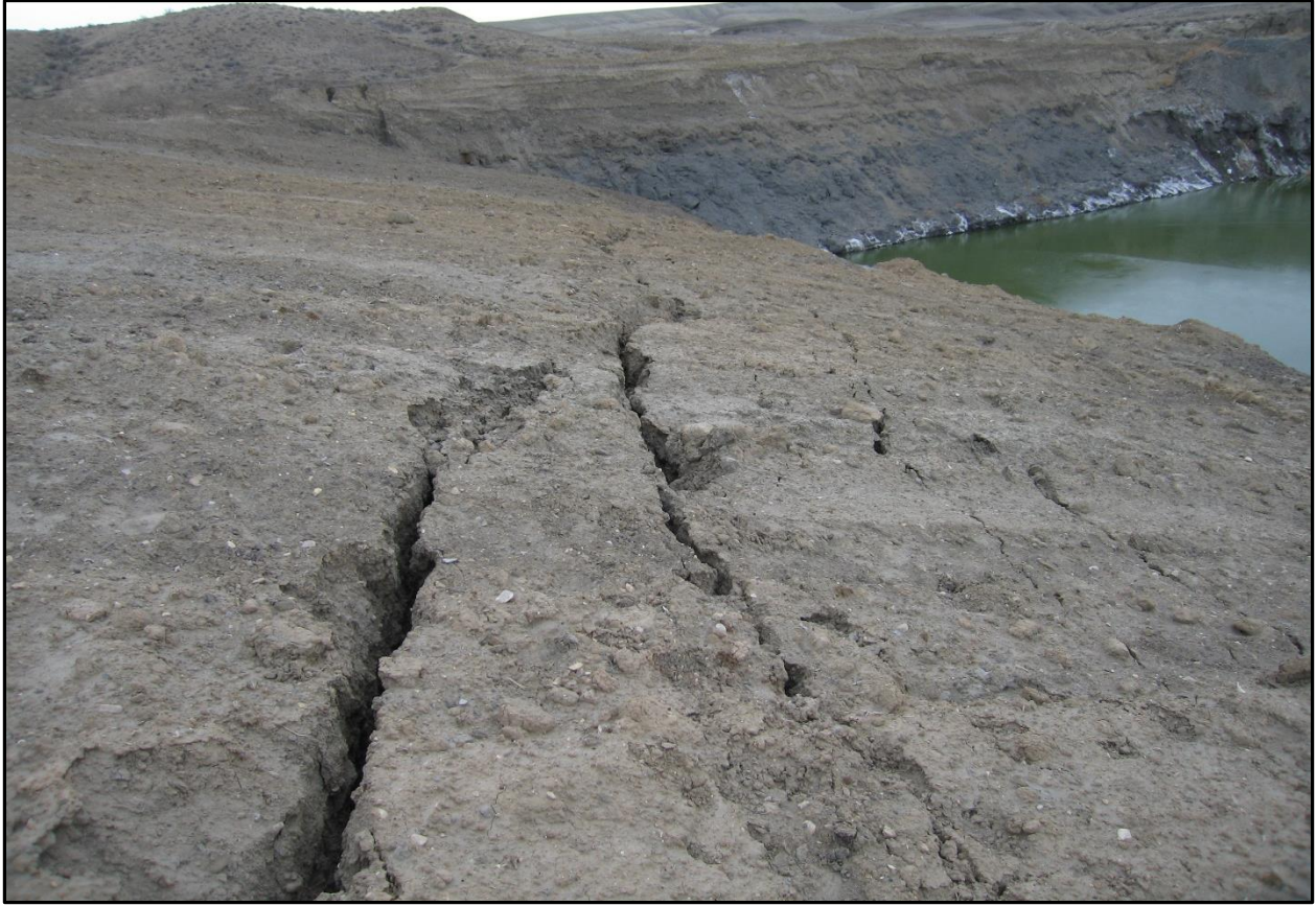
Photo 9 (above) looks north-northwest across a regrade area on the side of the north pond area where a series of tension cracks have developed. Photo 10 (below) is a close-up of a tension crack.
